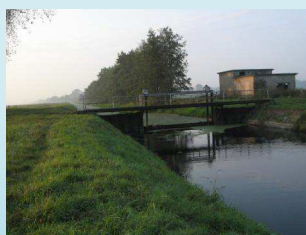
Wehr an Mündung in GHKK (BW1)
