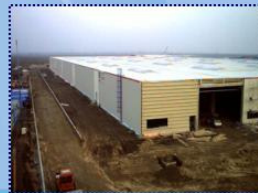
Yazaki Project Developed in "Crangul lui Bot" Industrial Park
