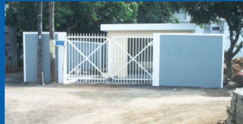
Pumpstation Grand Baie
