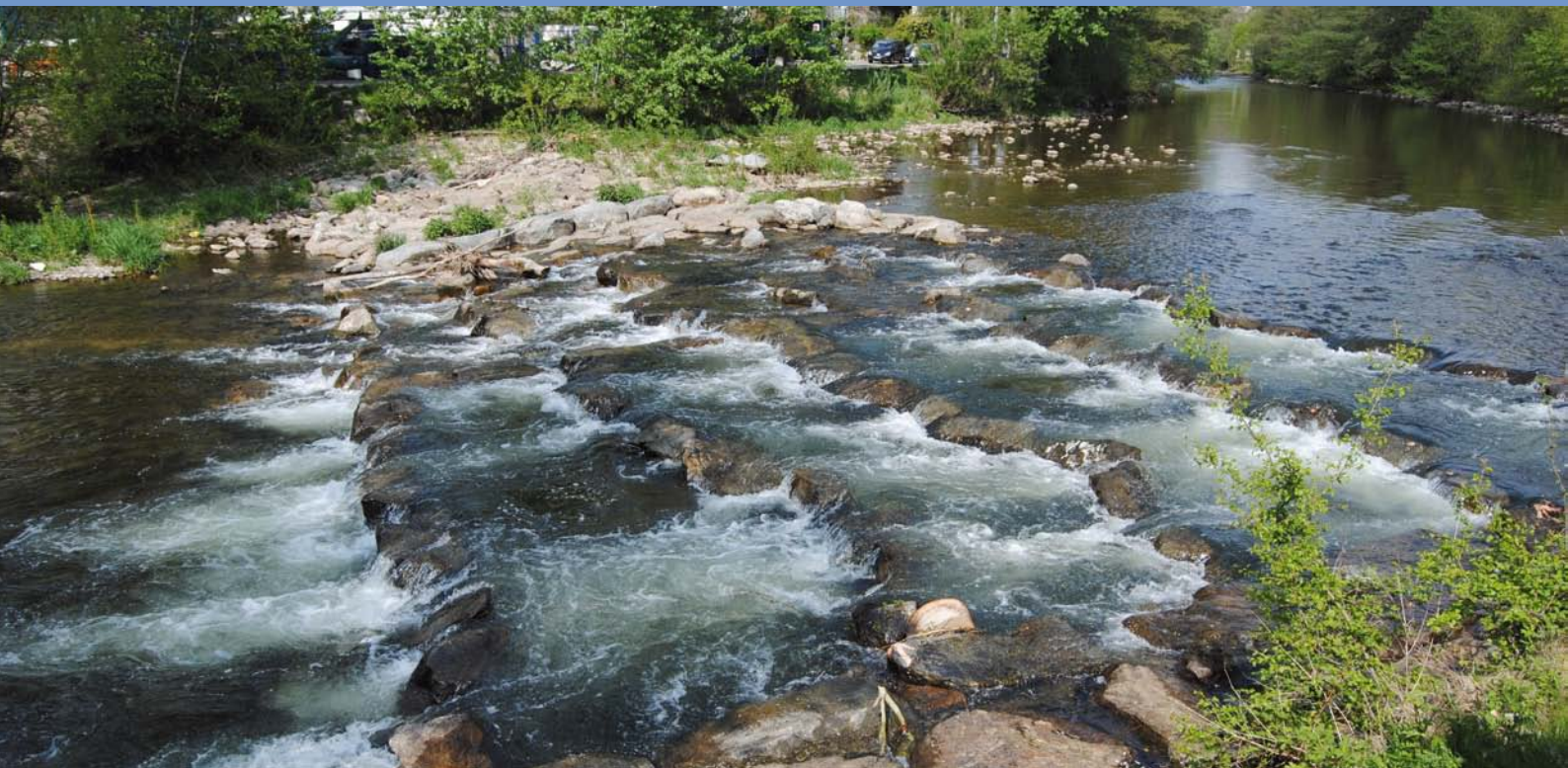
A former weir was redesigned as a river bottom ramp. Now fish and other aquatic organisms can pass this stretch again.
