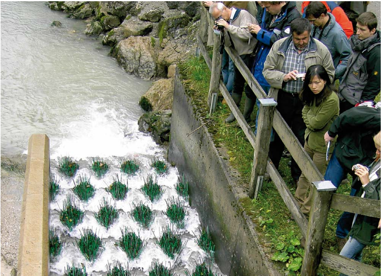
Bristle pass - another good means of ensuring the continuity of streams
